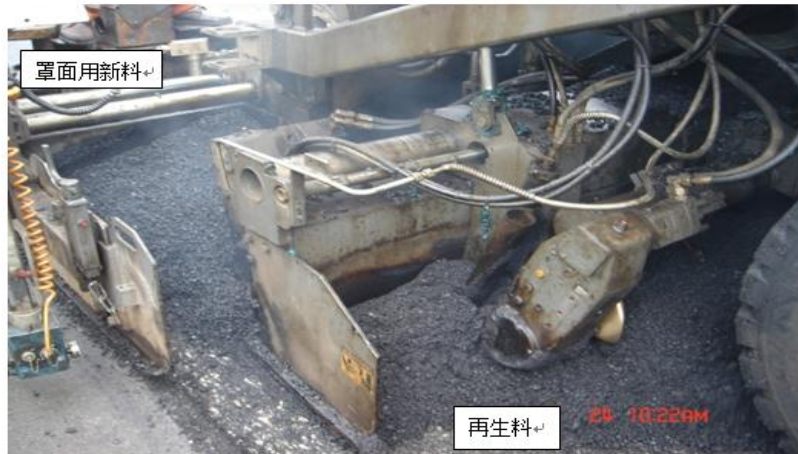
Fig 4. Tracking observation after hot-in place regeneration
