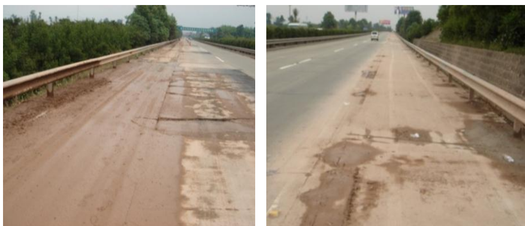
Fig 1. Original pavement condition
