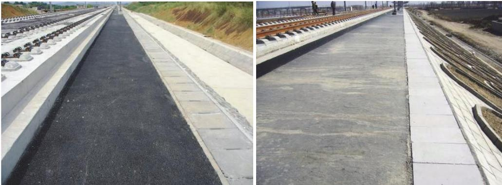
*Figure 6. RAC surface layer used in China*
