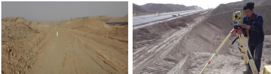
a) Measuring piles on site
