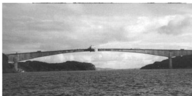
Figure 1. Stolma Bridge (Norway)
