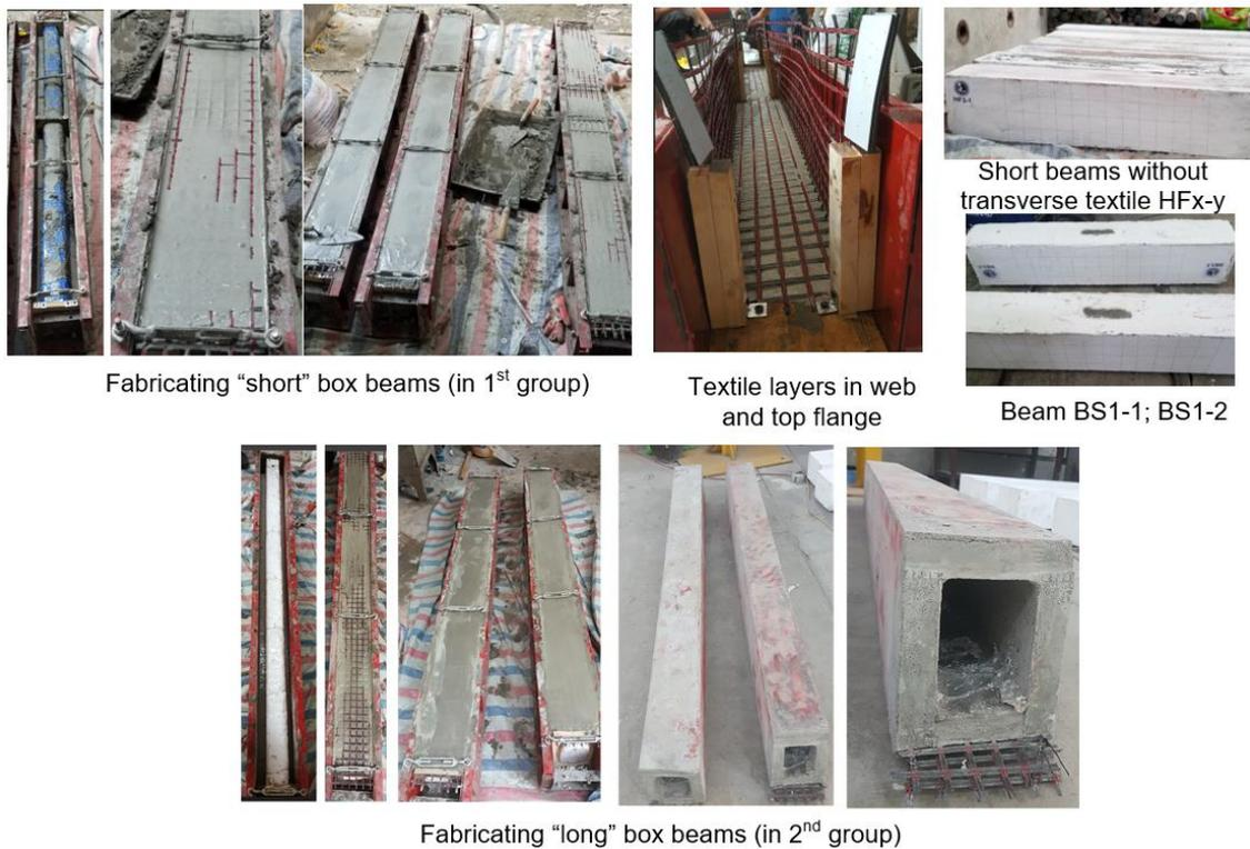
**Figure 4.** Fabricating ten box beams in two groups
