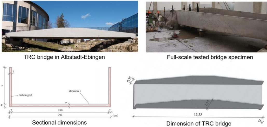
**Figure 1.** The first bridge made out of pure carbon concrete in Albstadt-Ebingen (Germany) [2]
